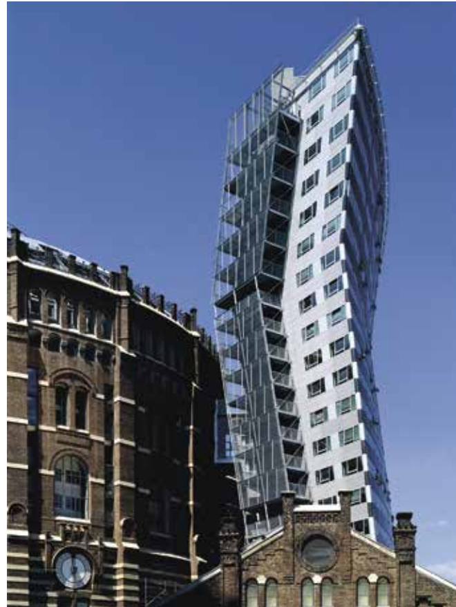
Gasometer, Vienna, Coop Himmelb(l)au, Photo: Gerald Zugmann
